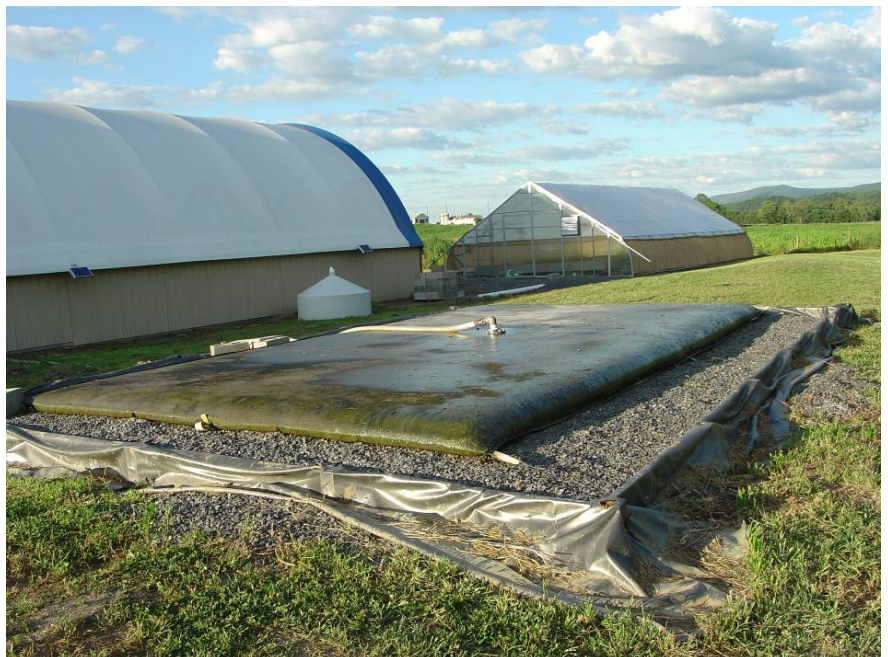
Photograph of Geotube at Reymann Memorial Farm
